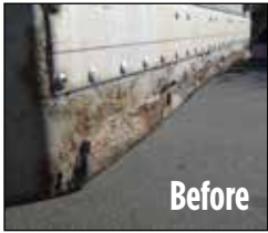
Repair and Paint Corroded Base Rails
